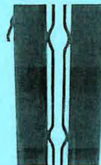
Integrated welded lacing rods
