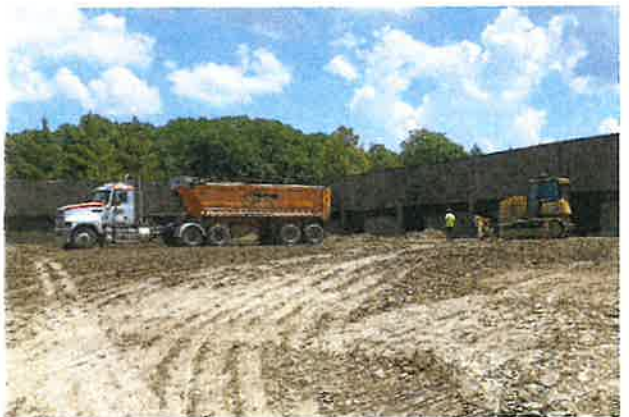
10 classroom building pad fill in progress
