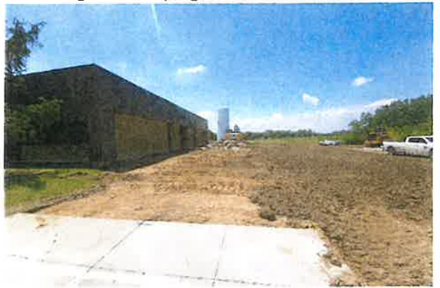
4 classroom building pad fill in progress
